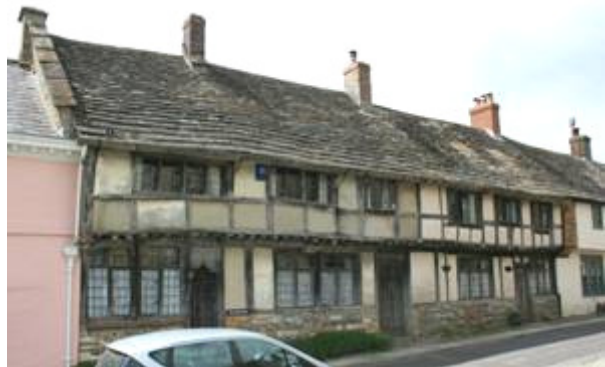
Figure 54: Abbey Cottage and the Pitchmarket; late medieval timber-framed tenements at 3-5 Abbey Street.
