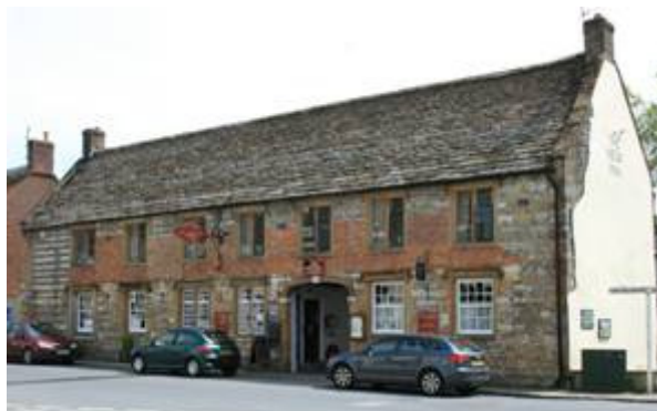
Figure 53: View of the New Inn, Long Street..
