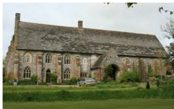
Figure 10: View of the Tithe Barn from the east.
