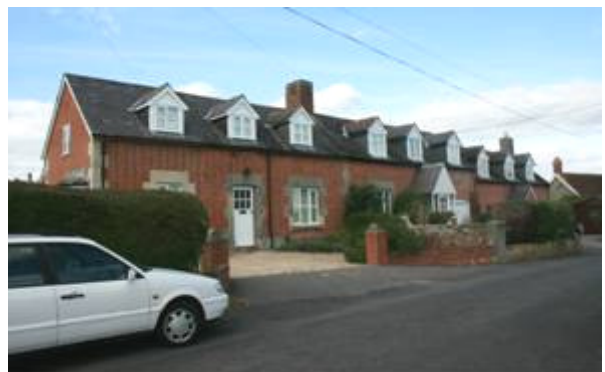
Figure 117: Terraced houses, 8-12 Breach Lane.
