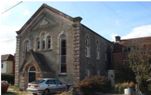
Figure 120: Former Methodist Chapel, Breach Lane.
