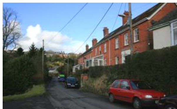
Figure 98: Edwardian Terraced Houses, Layton Lane.
