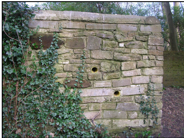
Plate 9. Wall B showing varied construction/repair materials
