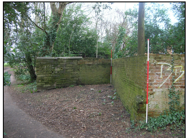
Plate 10. Wall B showing change from stone to red brick construction
