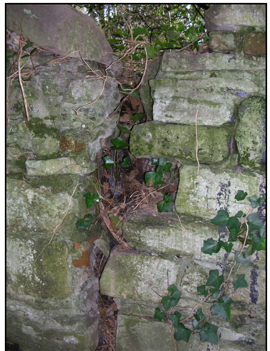
Plate 7. Crack in Wall B showing limestone facing with ironstone/heathstone core
