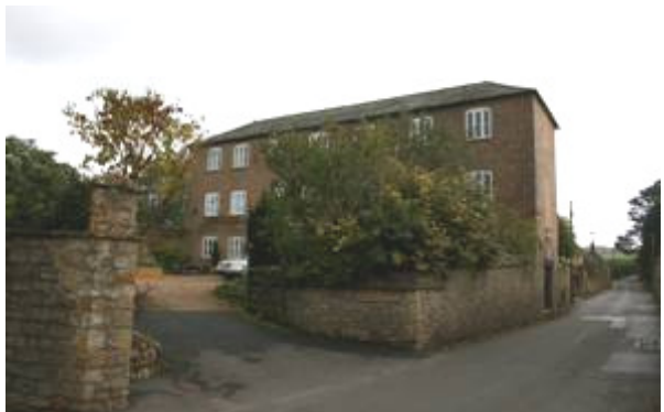
Figure 63: Flax Mill House, Whitcombe Road, a former industrial building.
