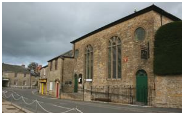
Figure 67: Former Congregational Chapel, Whitcombe Road.
