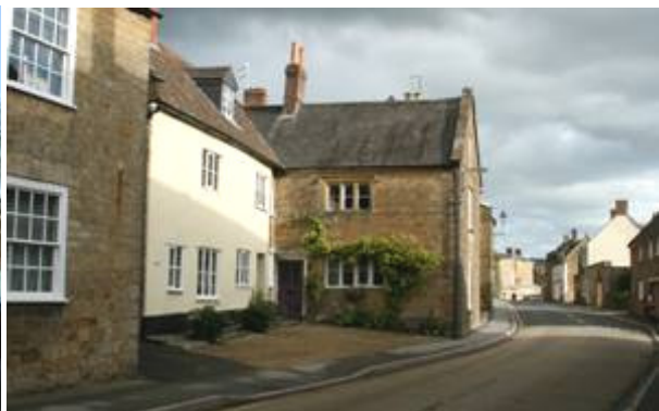
Figure 10: 17th century house at 56 Hogshill Street.
