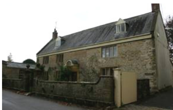
Figure 13: The 17th century 'Hitts House' Whitcombe Road.
