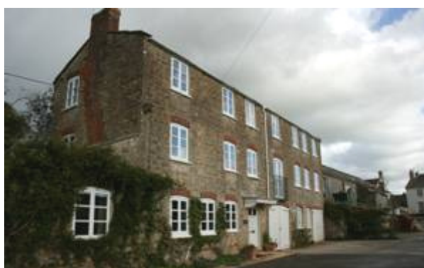
Figure 15: Former twine manufactory, Shadrack Street.
