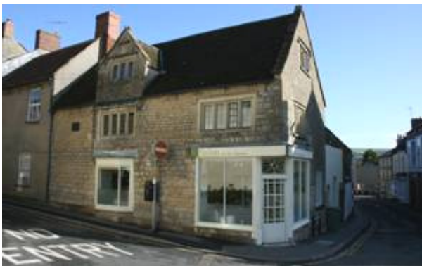
Figure 14: 12 The Square, built 1687 after the 1684 fire.
