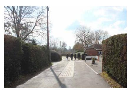
Central drainage channel to a road allows for the edges to be used by pedestrians and cyclists without obstruction.
