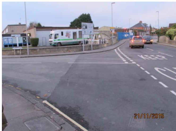
Brinsley Close showing lack of dropped kerbs and excessive road width
