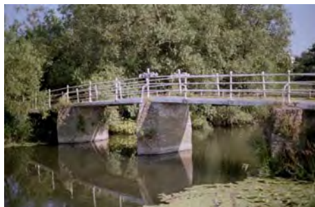
Figure 4: Colber Bridge over the River Stour
