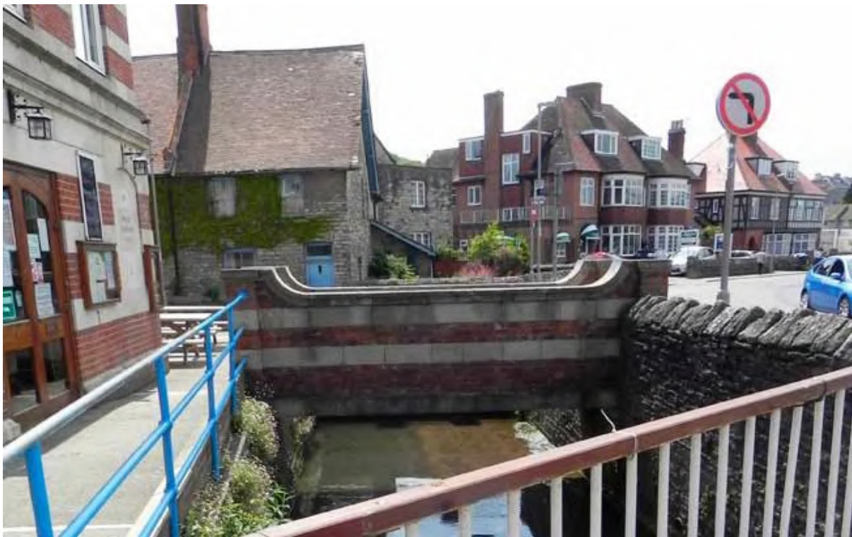
The Swan Brook outside the main Post Office is contained in channel and is culverted under Station Road re-emerging adjacent to the Mowlem
