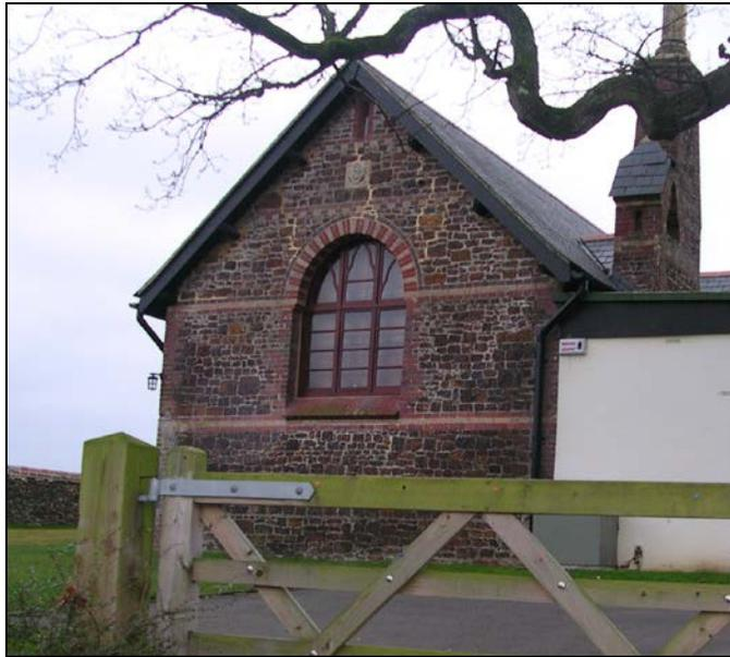
*Heathstone construction. Above Left: found as a component of flint and limestone walling in Winfrith. Above Right: Used as a principal material in construction at East Lulworth.*
