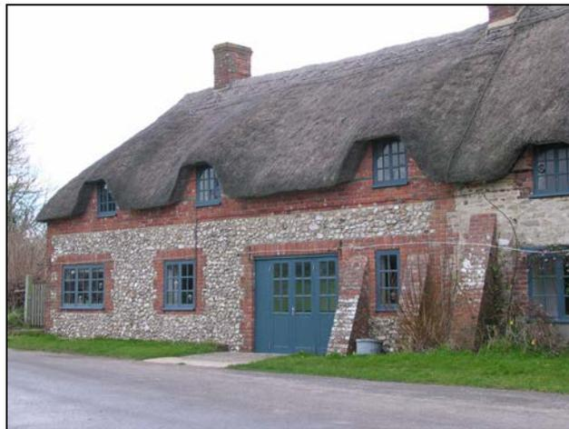
*Flint walls. Left: field flints employed in a boundary wall at Winfrith. Right: Cottage walling with brickwork forming openings and corners at East Chaldon.*
