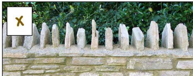
*Coping stones should bridge the width of the wall and be laid with no gaps between. Top left: rough cock and hen, typical of informal traditional building and the flank or garden walls of Edwardian properties. Top right: tightly packed, shaped stones in 'cock and hen' sequence, a finish typically seen on the front boundary walls of Edwardian properties in Swanage. Bottom: random shards of stone set in mortar and widely spaced.*
