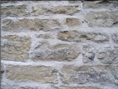
*Well coloured, textured lime mortar is finished flush between the faces of adjoining stones. See Appendix 2 for sample repointing method statement.*
