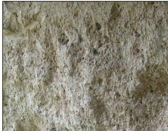
*Cob is normally given a protective render. The eroded cob on the right appears to contain some chalky subsoil.*
