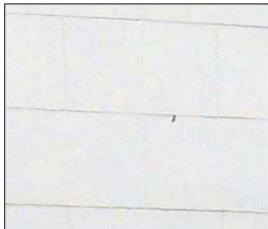
*Lined stucco in Wareham. The lines tend to become faint over time due to overpainting.*
