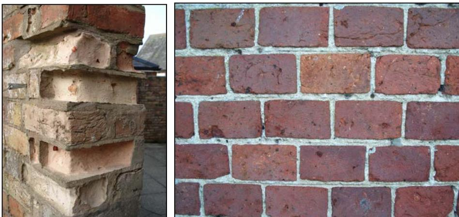
*Left: the catastrophic effect of pointing soft brick with hard cement mortar. Right: 'penny struck' pointing in header bond at Wareham. A finish in which the face of the joint has been scored using a penny.*
