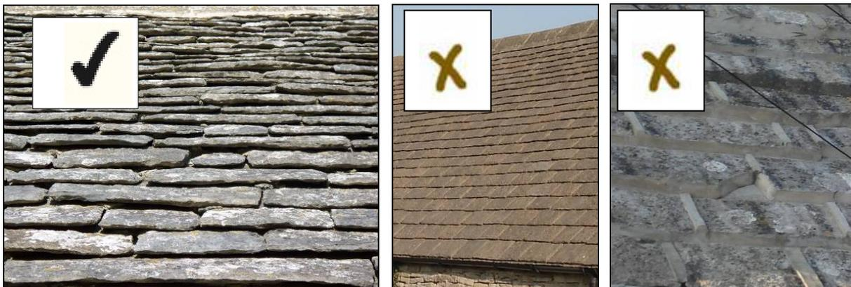
*Traditional stone roofing (left), artificial stone (centre), pointed roof (right).*
