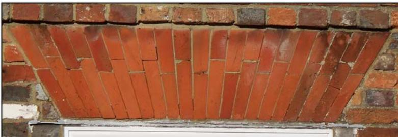
*Top: simple classical detailing arranged using specials, a soldier course (bricks on end) and rows of headers. Bottom: a Georgian gauged brick arch made using finely jointed 'red rubber' bricks.*
