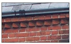
Left: moulded cornice detail. The outward kick of the roof slope has been achieved by 'spocketting' the eaves. Note the rise and fall gutters held on brackets. Right: dog tooth detailing with an 'ogee' profile box gutter.
