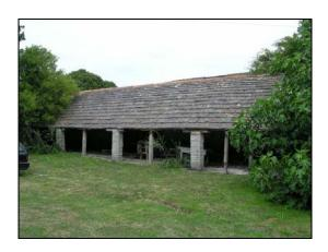
Shelter shed (Barnston). Three bays shown, the roof of which is propped. Bays are wider and roof lower than would be found in a cart shed.
