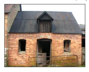
Small brick stable with corrugated roof. Note the internal shutters on the windows – a common means of window closure on agricultural buildings generally which were rarely historically glazed.
