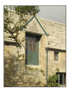
Door changed to window. Whilst this loading door is no longer in any active use, its identity as a door has been retained whilst its function has changed to that of a window. This approach may not be appropriate in every case, but the principle is well illustrated in this photo.
