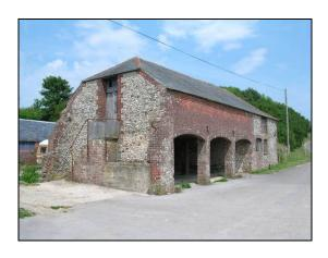
Flint and brick cart shed with granary over (West Lulworth). External steps serve the latter. A small stable which extends to the rear fills the fourth bay.
