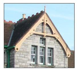
Left: bargeboard detail. Note the moulding on the upper edge. (Swanage). Right: bargeboard with finial extended through to a strut and collar. (Corfe Castle). Such bargeboards form part of an overall stylistic package and provide considerable visual interest.
