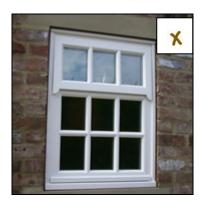
Top hung plastic window which crudely imitates a traditional sash window. Detailing, opening mechanism, materials and fitting are poor. Genuine sliding sash windows with this configuration were typically 'single hung' i.e. the top panel was fixed. Note the horns, not traditionally employed on multi-paned windows, the thick meeting rail and chunky glazing bars.
