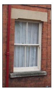
Left: Flush fit multi-paned sash window with exposed box in Wareham. Right: sash window with recessed box and reveal in Wareham. Centre: cross section through a sash window.
