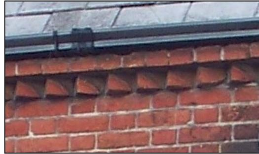
*Left: moulded cornice detail. The outward kick of the roof slope has been achieved by 'spocketting' the eaves. Note the rise and fall gutters held on brackets. Right: dog tooth detailing with an 'ogee' profile box gutter.*
