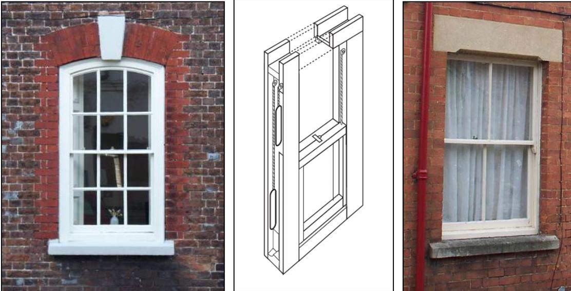
*Left: Flush fit multi-paned sash window with exposed box in Wareham. Right: sash window with recessed box and reveal in Wareham. Centre: cross section through a sash window.*
