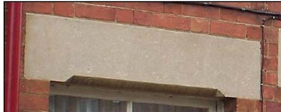
*Arches and lintels. Top left: a finely jointed gauged brick 'flat' arch (Wareham). Top right: timber lintel (Corfe Castle). Bottom left: stone arch – more common in brick (Corfe Castle). Bottom right: stone lintel with chamfered edge (Wareham).*
