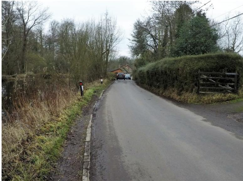
By the Sheep Wash area between No. 33 and The Old Rectory bridge, continued use of the verge has damaged the road edge and created a hazardous drop – *See attached picture:*
