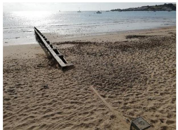
Figure 3-6 Photos showing 4m gap in the waling beam towards the landward end of each timber groyne, so allow access along the beach.
