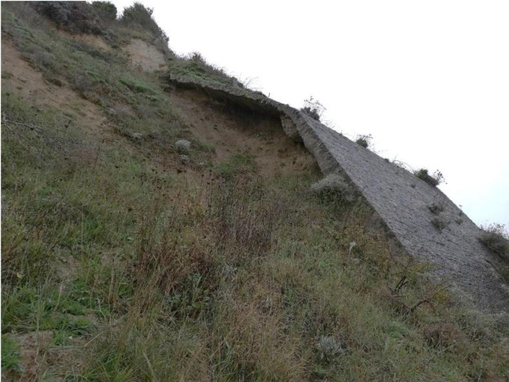
*Figure 3-10 An example of historic ad hoc slope stabilisation measures introduced along the New Swanage frontage by a private landowner (photo taken on 24<sup>th</sup> October 2019).*
