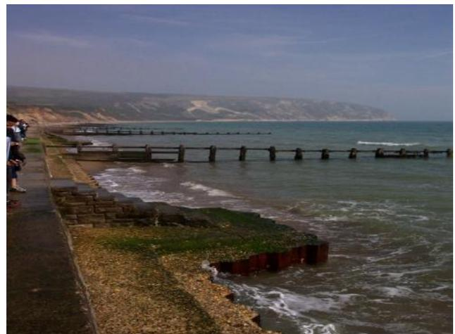
Figure 3-9 Parts of the seawall along the New Swanage frontage refurbished/rebuilt in 1962, with steel sheet pile exposed when beach levels were lower, prior to beach recharge in 2005 (left = from Goater, 2014; right = from Royal Geographical Society, 2007).
