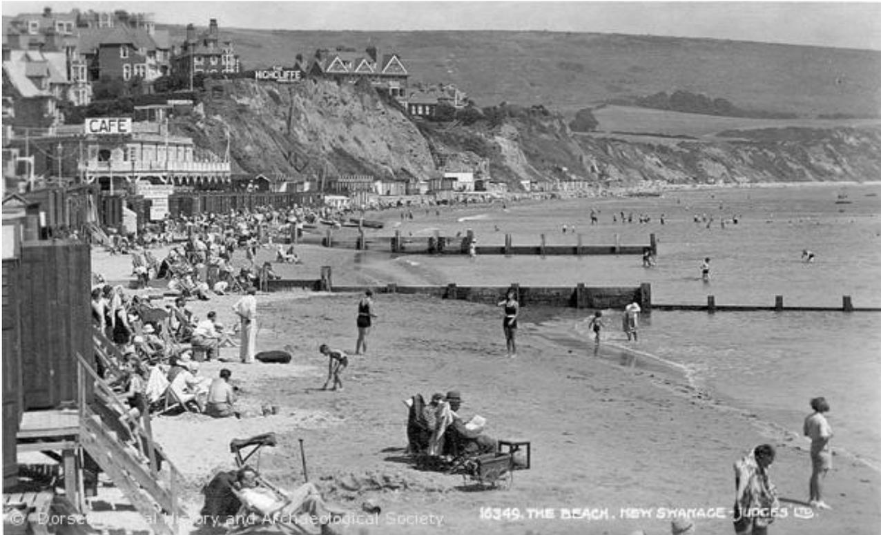
Figure 1-5 Photo showing the older timber groynes along the Shore Road part of the BMP frontage, prior to construction of additional timber groynes northwards along the New Swanage frontage. Date thought to be around 1949. Photo from Channel Coastal Observatory. Owned by Dorset County Museum. Copyright Dorset Natural History and Archaeological Society.
