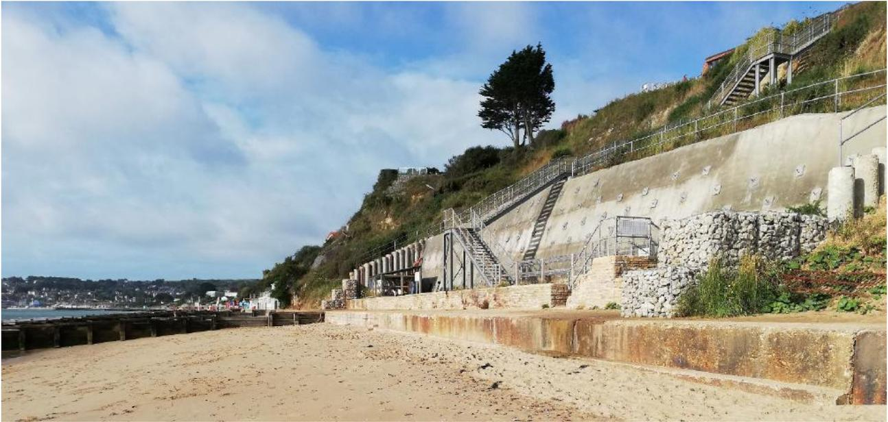
Figure 3-11 The Pines Hotel slope stabilisation scheme constructed by the private landowner between 2015 and 2017. The 1960s seawall and 2005 timber groynes at the base of the cliff are also shown.
