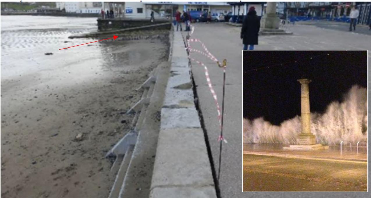
Figure 1-4 Significant damage occurred to the seawall along Swanage promenade between the Mowlem and the Banjo Pier as a result of a storm on 14<sup>th</sup> February 2014. This displaced approximately 25m of top stones (from JBA, 2020a). Note also an exposed, historic rock groyne-type structure adjacent to the slipway (marked with an arrow). Insert is a photo of waves breaking on the seawall during the same storm event (from Goater, 2014).
