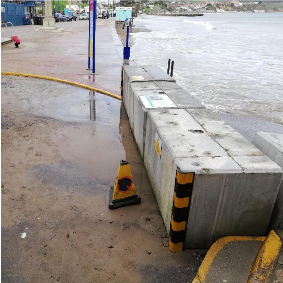
Figure 4-4 Seasonal concrete wave barriers installed at the top of the slipway adjacent to The Mowlem at the southern end of the BMP frontage in February 2020.
