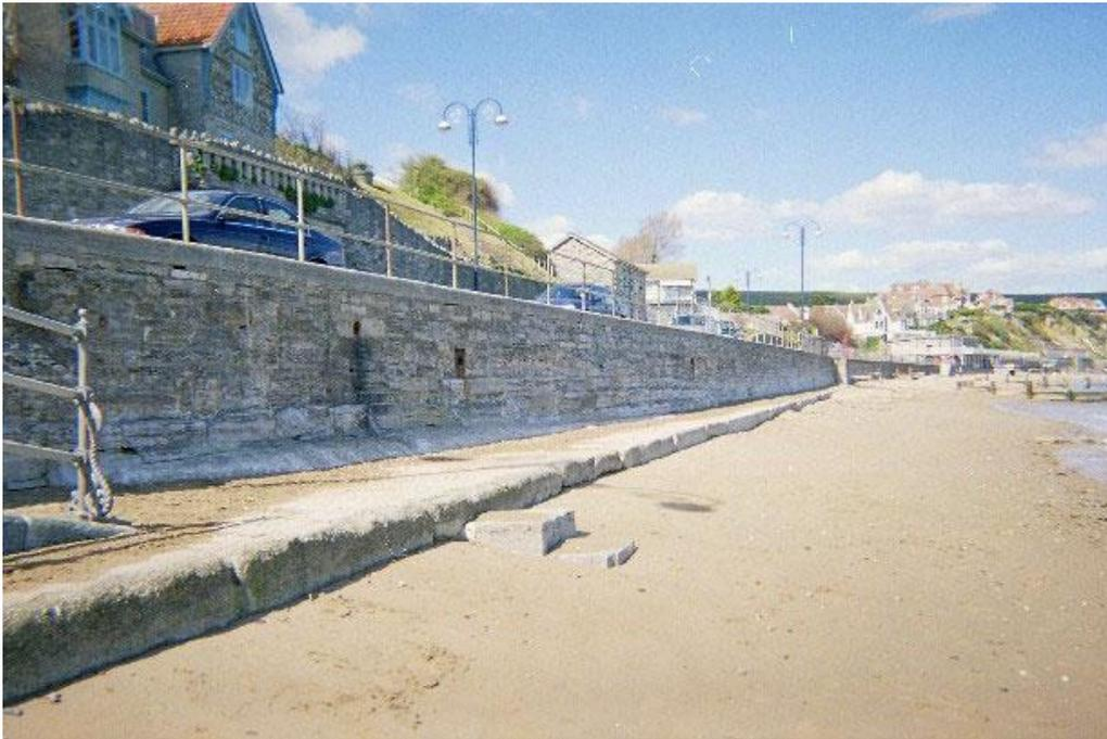
Figure 3-8 1920s seawall along part of Shore Road exposed by low beach levels prior to beach recharge in 2005, shows toe details (from Goater, 2014).
