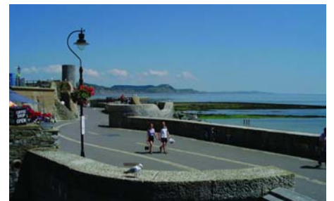
Phase 1 works provided a new promenade for the town.
