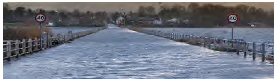
Figure 12 Flooding of South Causeway 2014
