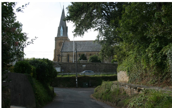
Figure 138: View of Holy Trinity Church from Middle Street, Bradpole.
