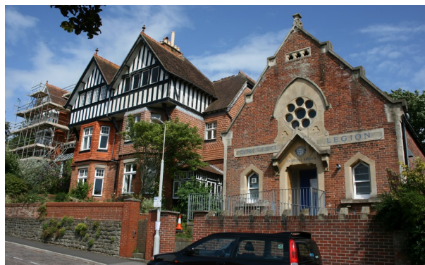
Figure 126: British Legion Hall with 48-50 Victoria Grove adjacent and No. 52 in background.
