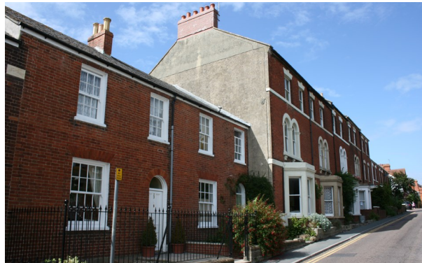
Figure 127: 23 and 25 Victoria Grove with the three-storey 27-37 Victoria Grove behind.
