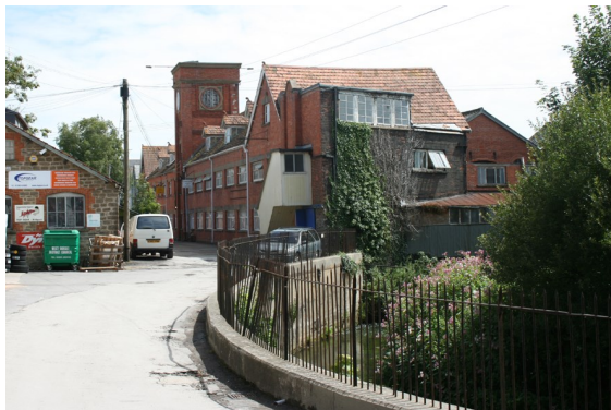
Figure 34: 'Bridport Industries' Building, St Michael's Lane.
