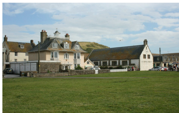
Figure 33: 'The Moorings' and St John's Church, West Bay.
