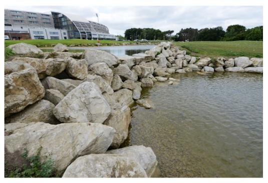
various contractors, including Keltbray and Maccaferri, 850 tonnes of ½ to 2t Rock, 550 tonnes of gabion stone and another 145 tonnes of auxiliary stone gradings were supplied by Suttle Stone Quarries to achieve spectacular views over the landscape and stadium walls. The work was
