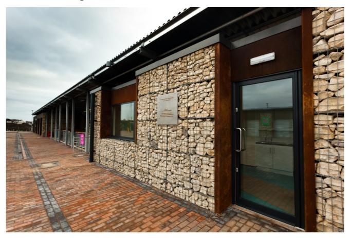
Suttle Stone Quarries, provided 100-200mm Gabion Limestone for filling Gabion Basket retaining walls at the new household recycling depot in Swanage for work completed by Raymond Brown Construction for Dorset County Council in 2012.
