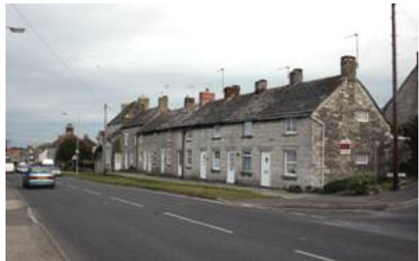
Figure 129: Purbeck Stone cottages along High Street.
