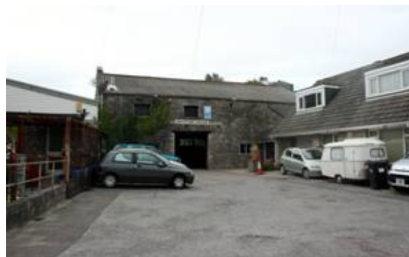
Figure 100: Part of former gas works.
