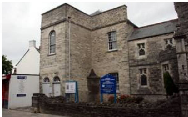
Figure 15: Congregational Chapel, built 1837.
