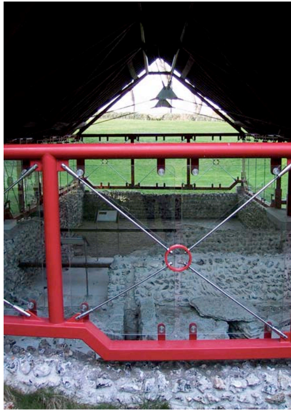
View looking north through gable end of Room 17, illustrating the stainless steel fixings on the glass panels.
