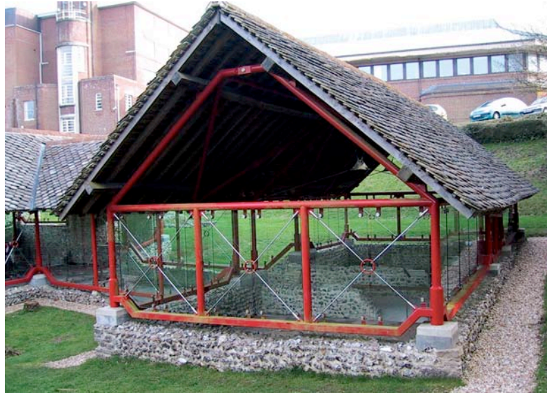
Room 18 - exterior, gable end. This plate illustrates the huge unprotected area of the gable ends of the cover structure, allowing wind, rain, birds etc to enter the building.
