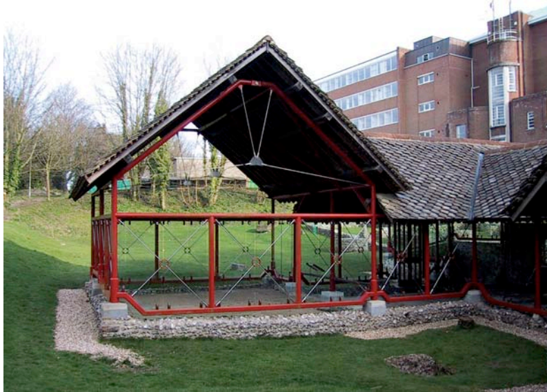
Room 15 - exterior, gable end. This plate illustrates the huge unprotected area of the gable ends of the cover structure allowing wind, rain, birds etc to enter the building.
