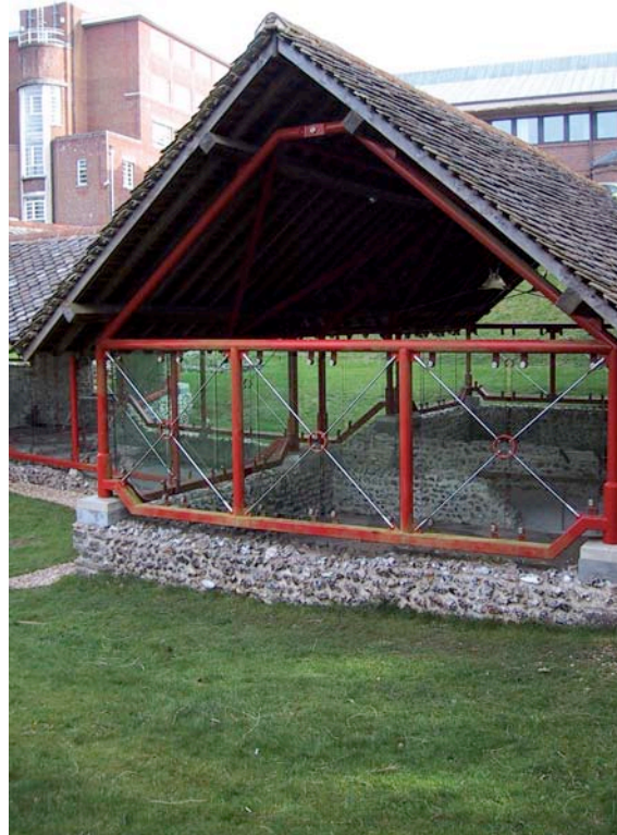
Room 18 - exterior, gable end. This plate illustrates the huge unprotected area of the gable ends of the cover structure, allowing wind, rain, birds etc to enter the building.
