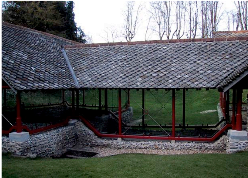
Room 13 (and corner of Room 17) - Uneven tiles. This plate illustrates the fixing of the roof tiles, which, because they have not been attached in the original Roman manner and no other weather proofing has been provided (roof felt etc) allows wind blown rain to penetrate.
