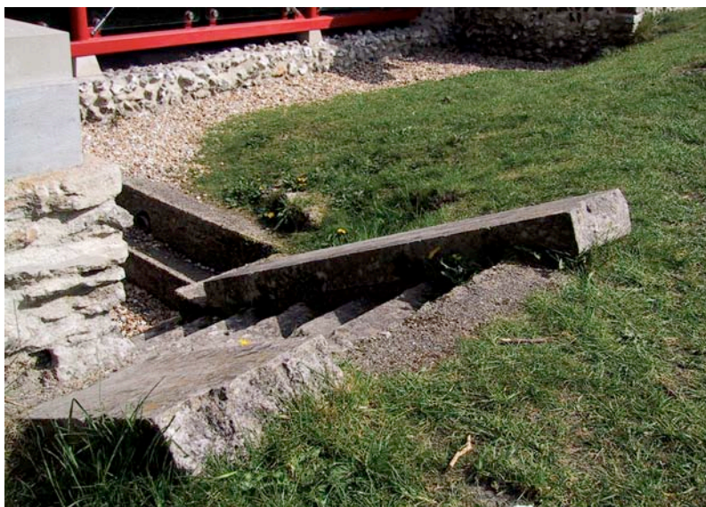
Room 17 – exterior steps at 17a. The tops of these steps pose a possible safety hazard to visitors as they protrude above ground level. Thought should be given to the provision of a safety rail.
