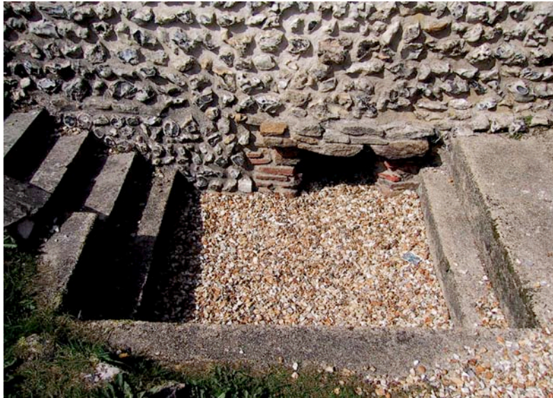
Room 17 – exterior hypocaust stoke hole (17a). This open hole is used by both animals and humans to gain unauthorized entrance to the building. It should be closed with fine metal mesh.
