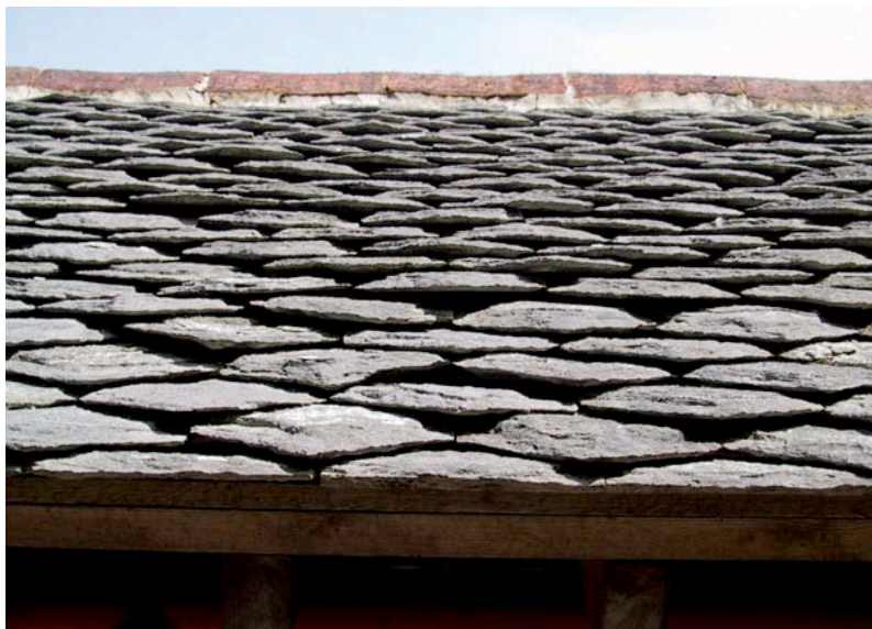
Room 13 -Uneven tiles. This plate illustrates the fixing of the roof tiles, which, because they have not been attached in the original Roman manner and no other weather proofing has been provided (roof felt etc) allows wind blown rain to penetrate. Close up.
