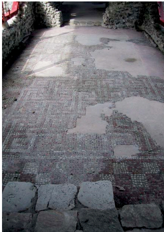
Room 13 - mosaics open to the public! This area is at present open to the public and is the main walkway from the entrance to view Rooms 16, 17, and 18. The southern side has a rope barrier directing visitors to walk on the northern side which is damaging the mosaics in this area. Increased traffic and contra-flow exasperates the problem. Note acute sunlight, shadow and damp patches. Steps from Room 10 to 13 are unsuitable for less-abled.
