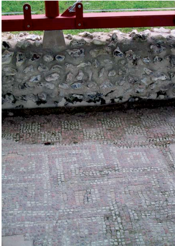
Room 13 – South wall. Damp. This plate shows the effects of water that drips down from the top of the Roman walls on to the mosaic floor
