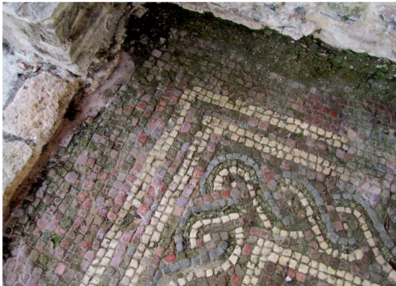
Room 10 – SE corner near window. Showing effects of damp and algae
