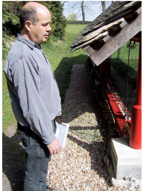
Room 17 - SW corner. Illustrating the relative adult height to corner roof overhang. This is a severe danger.
