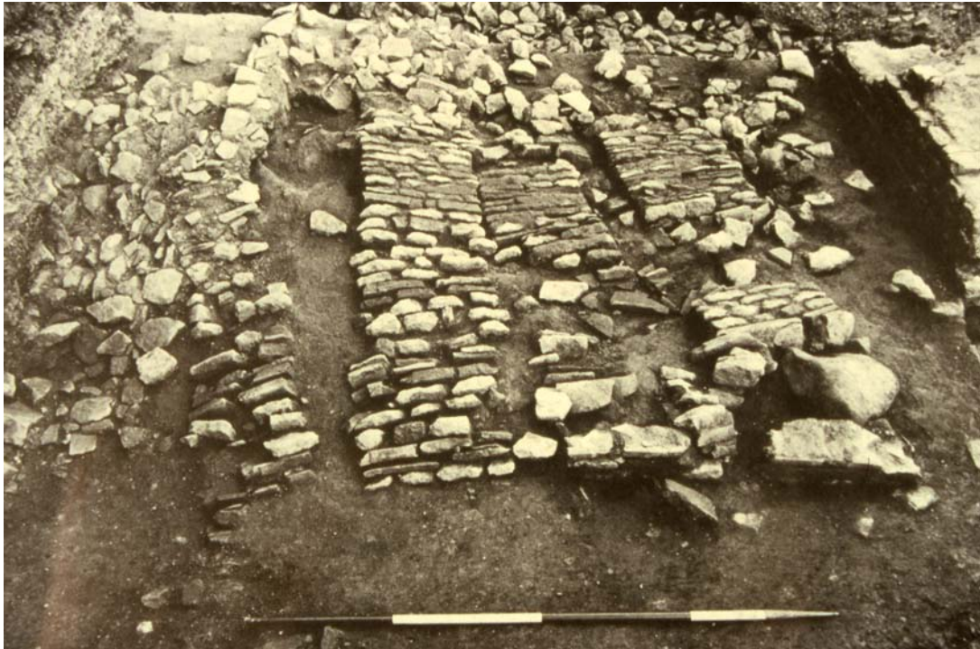
Plate 15. Collapsed internal wall from a 2 nd century building at Cirencester. The wall was timber framed and infilled with masonry. The estimated height of the wall is 3.1m. (From Holbrook 1998).
