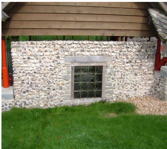
Plate 14. Room 10 window re-erected and as displayed prior to 1996 (left); as restored 1999 (right). The iron grille is based on an example discovered at the Hinton St Mary villa in Dorset.
