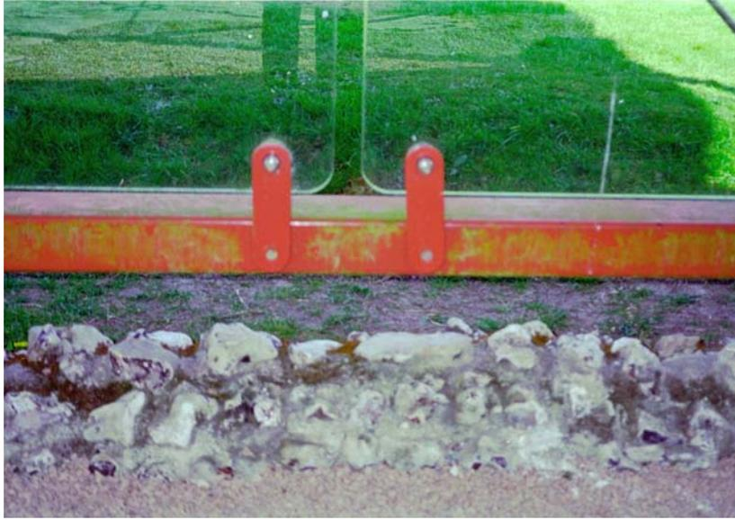
Plate 5. Room 15. Steel-frame structure with glass panels. Note: algae on horizontal frame and the gap between frame and wall.
