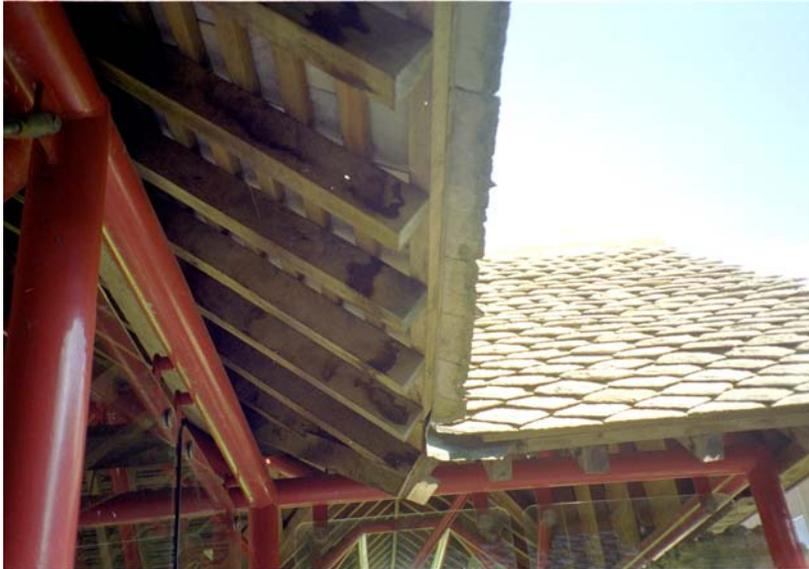
Plate 6. Cover building, South side, under eaves,. Note: stains on wooden roof supports
