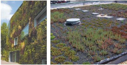
Enhancing the existing building with green walls and roofs
