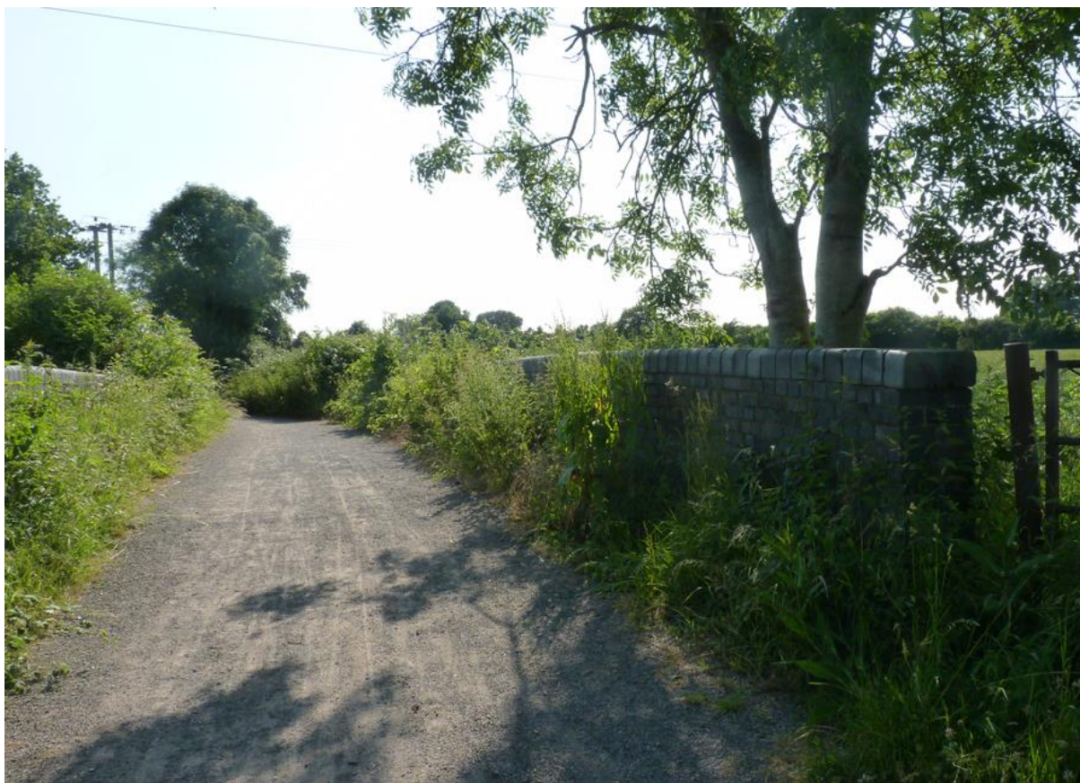
Figure 7.17: Ward’s Drove Bridge, looking south-west along Ward’s Drove
