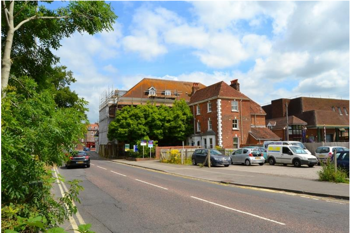
Figure 7.10: View north along the road into Blandford Forum showing Magnolia Court with a vacant area used for car parking in the foreground and Morrisons Supermarket far right
