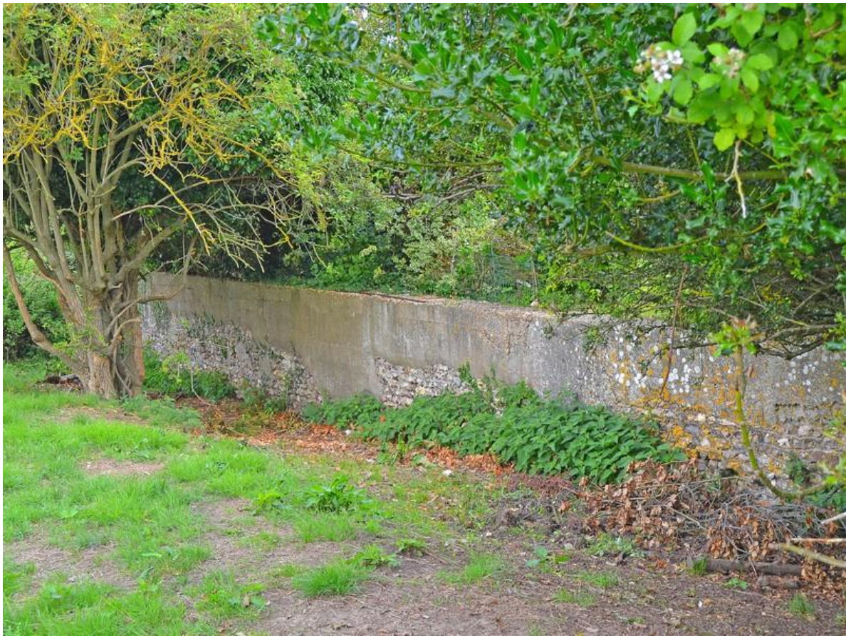
Figure 7.23: Detail of the anti-tank ditch with the ha-ha wall set into the ground to maintain visibility across the structure
