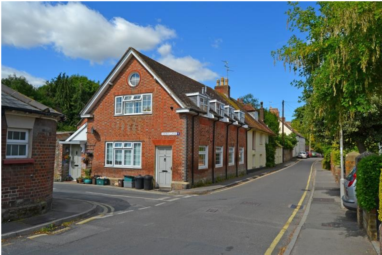
Figure 7.15: This view looking west along Bryanston Street from the entrance to Short's Lane includes the street frontages of the listed properties Bethune and Bryanston Cottage
