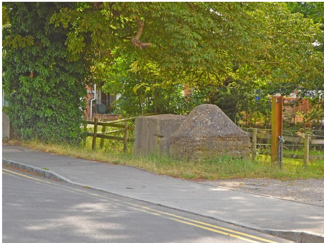
Figure 7.21: Concrete anti-tank cube and concrete 'dragon tooth' (cube with a pyramidal cap) on the south side of River Mews
