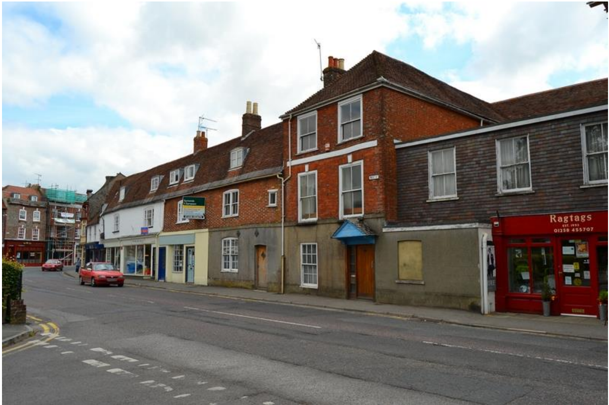
Figure 7.11: Buildings on the east side of West Street opposite the entrance to River Mews, showing the 3-storey Masonic Hall with 19 – 25 West Street beyond
