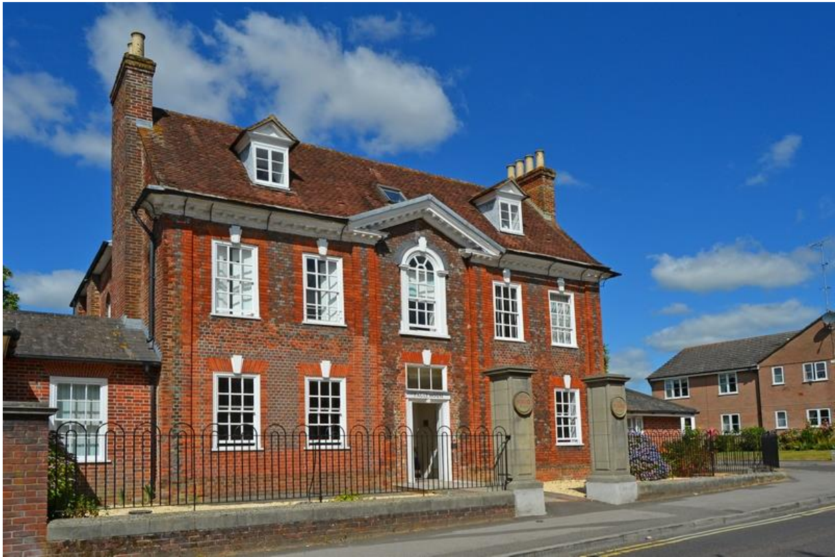
Figure 7.17: Eagle House, White Cliff Mill Street
