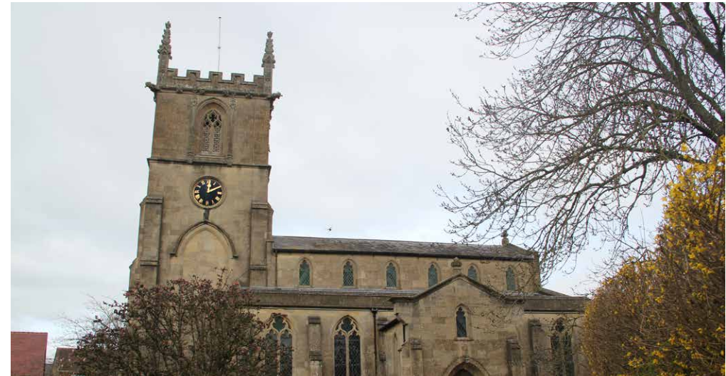
FIGURE 20. GRADE I LISTED CHURCH OF ST MARY
