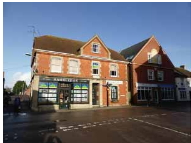
Melbury House and Phoenix House
