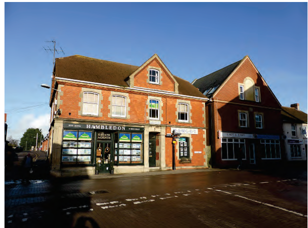
Melbury House and Phoenix House
