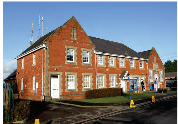
Town Hall and Police Station
