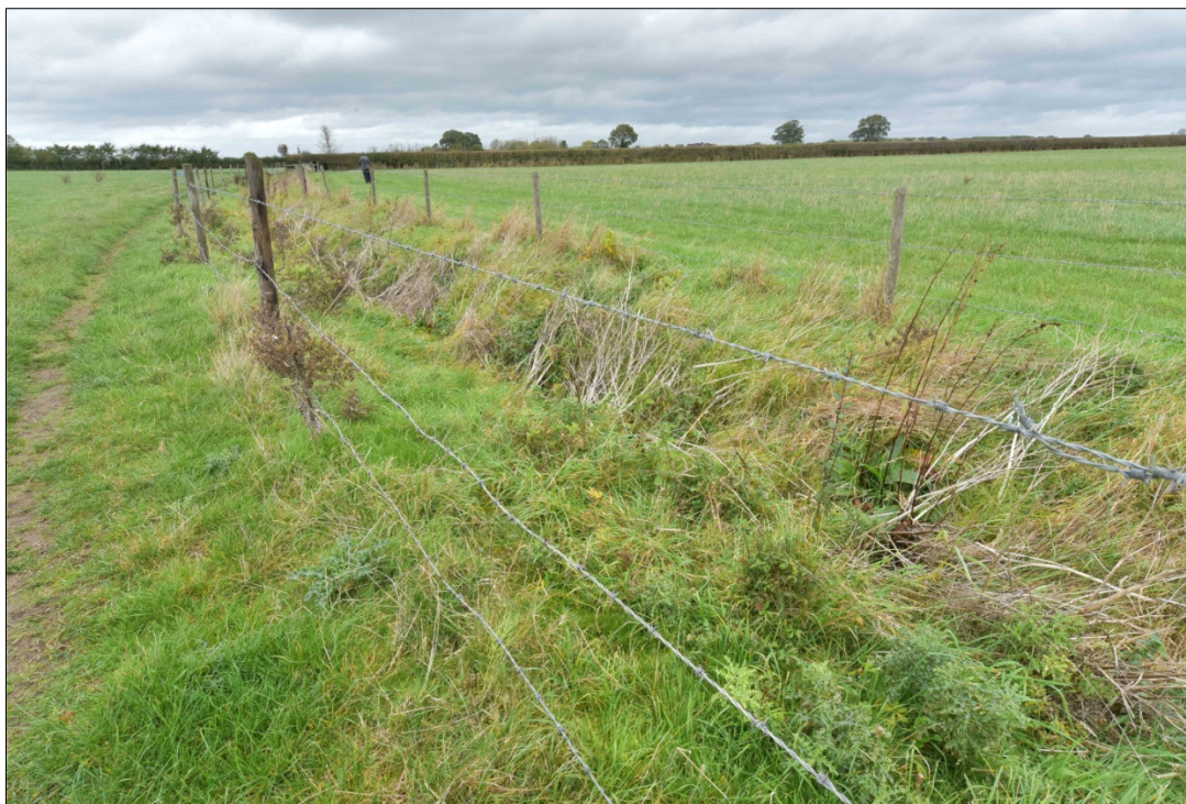
FIG 2. Field A, the fenced ditch which forms the eastern boundary.
