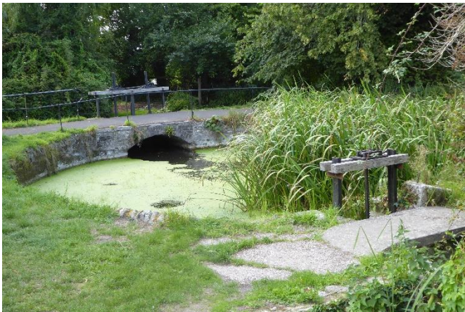
Examples of a bridge and sluice gate.
