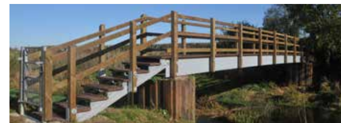
Refurbished footbridge in West Dorset improves pedestrian safety and supports active travel across rural infrastructure.
