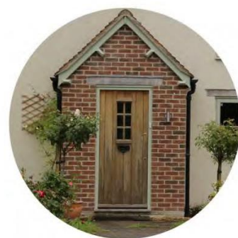
RED BRICK/TIMBER PORCH
