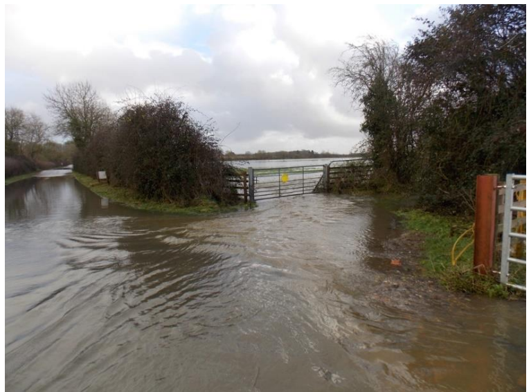
Figure 1. Flooding in Mill Lane from river overtopping
