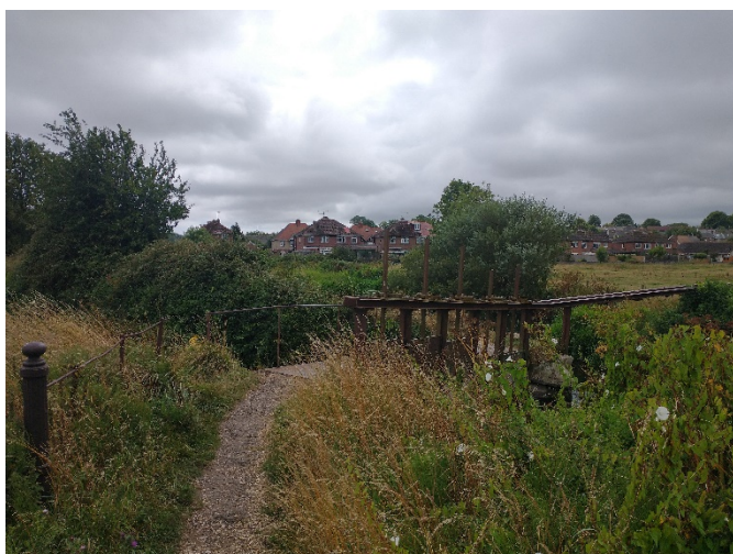
Figure 5.10: 'Ten Hatches Weir' near Grey's Bridge LUC ref: ND52
