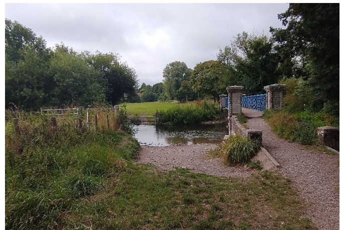
Figure 5.12: The 'Blue Bridge' [LUC ref: ND32] looking southwest
