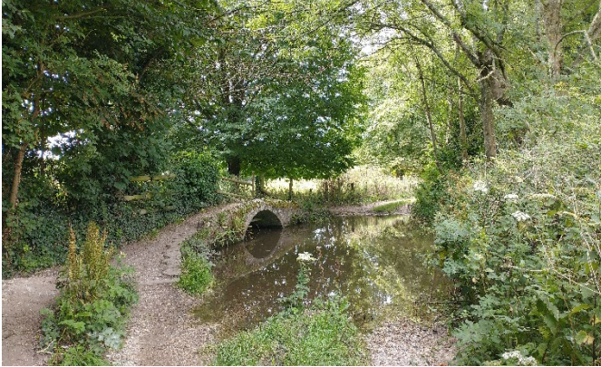
Figure 5.13: Footbridge east of Frome Whitfield House [LUC ref: ND39] looking south
