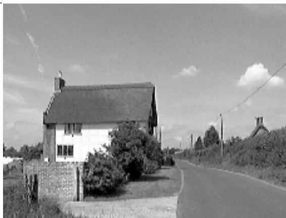
Court House, Cowgrove, an early 17th Century timber framed house, with wattle and daub panels, all treated with lime wash.
