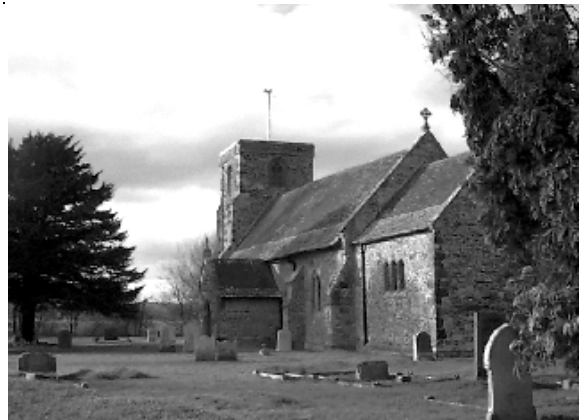
St. Bartholomew's Church, Shapwick, the nave and tower are mostly 14th Century, built onto an earlier structure. The walls are of flint and rubble with ashlar dressings. A mixture of Purbeck and heathstone is used, with Purbeck stone tiles on the roof eaves.
