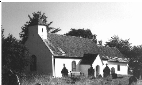
All Saints Church, Chalbury, partly refaced in brick, is now mostly rendered. Note the plain bell-cote on the west gable, and the stone eaves courses on the chancel roof.
