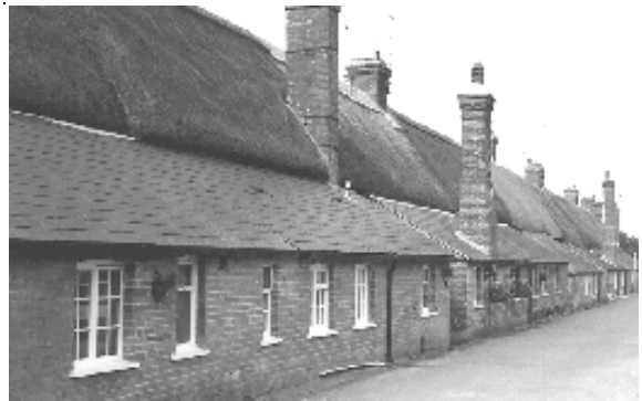
The Buildings at Manswood is reputed to be the longest continuous row of thatched houses in England. Note the rear slate roofed outshut and their tall chimneys.
