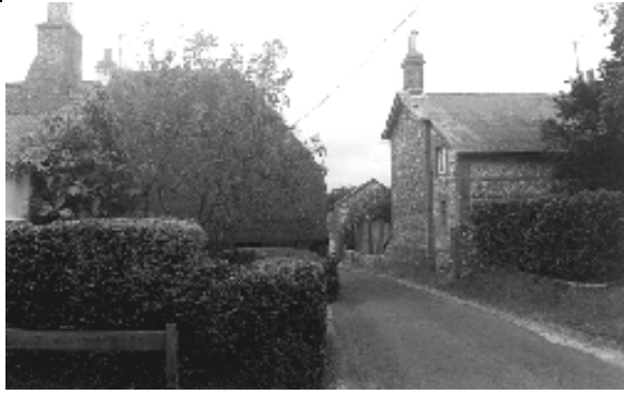
A narrow span two storey house in Woodyates; its low pitched slate roof extending at the rear to cover a two storey outshut. The walls are of flint, with brick quoins and horizontal bands.
