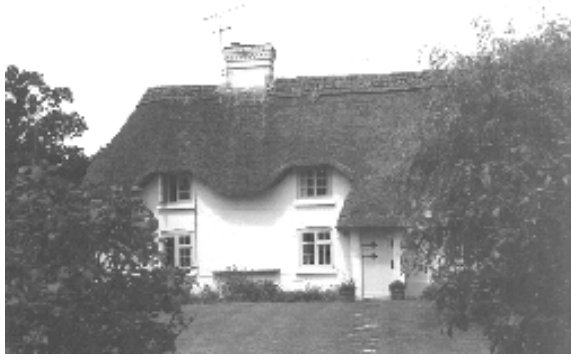
The scale and character of vernacular cottages derive from small rooms and low ceiling heights. Attic room windows are normally within 60cm. of the floor. Harkaway Cottage, Woodlands
