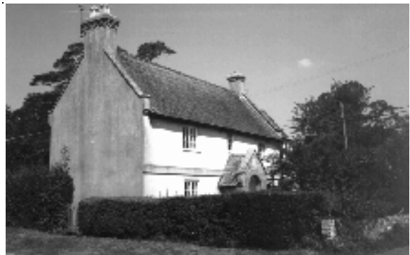
No.8 Village Street, Edmondsham fits the 'Small house' category, as defined by Brunskill. Note the alternating plain and fish-tail clay tiles on the roof and parapet gables. Identical stacks incorporated within each gable and symmetrical fenestration are common features of such buildings.
