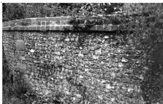
Coursed flint work with random ashlar pieces, capped with brick. Moor Crichel.
