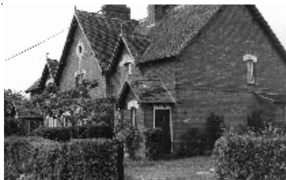
The design of many houses of this period followed one of a number of published pattern books. Though clearly contrasting from the earlier vernacular buildings, such houses are traditional in terms of their proportions and materials. In most instances only two or three were built in any single locality, in keeping with the area's slow organic growth. High Street, Shapwick.
