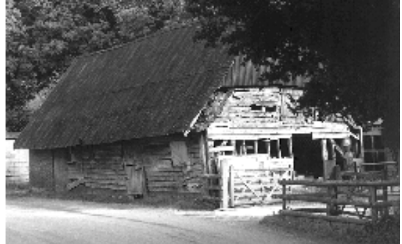
White Mill Farm barn, before restoration in 1998.
