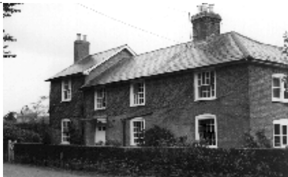
Brick represents the most common building material in the Stour valley, east of Wimborne. Manor Farmhouse, Hampreston.
