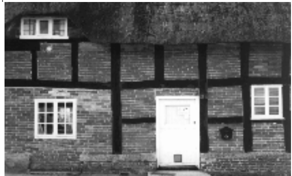
Square panels and straight braces characterise East Dorset timber frame buildings. Vicarage Farm, Holt.
