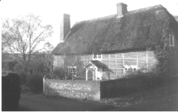
The basic form of the vernacular cottage, such as building width and roof height, is generally consistent, but a variety of features makes each one unique, Elm Tree Cottage, Gussage All Saints, features a single gable and half hip and irregular fenestration pattern.
