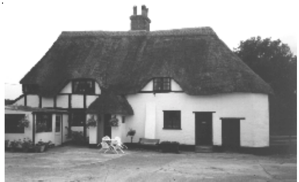
Hart's Farm, Horton, a single storey with attics timber frame 17th Century house, part re-faced in brickwork in the 18th Century.
