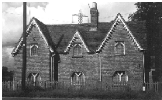
Owners have a responsibility to preserve the character of interesting old buildings: retaining timber windows, decorative barge boards, tiled roofs and tall stacks. Estate houses near the Grange, Furzehill.
