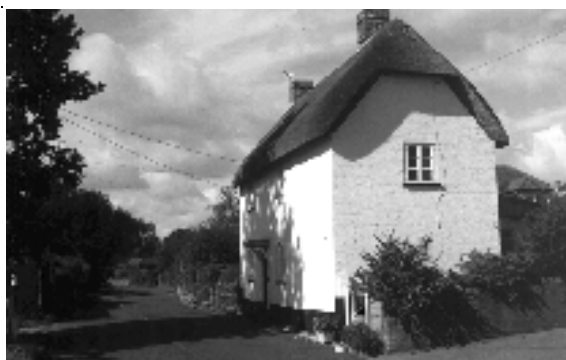
Thatch was still used in East Dorset as late as the 19th Century. For example, Trafalgar Cottage, Back Lane, Sturminster Marshall, has rendered walls, which are of rubble, above a brick plinth, perhaps recycling materials from an earlier building.
