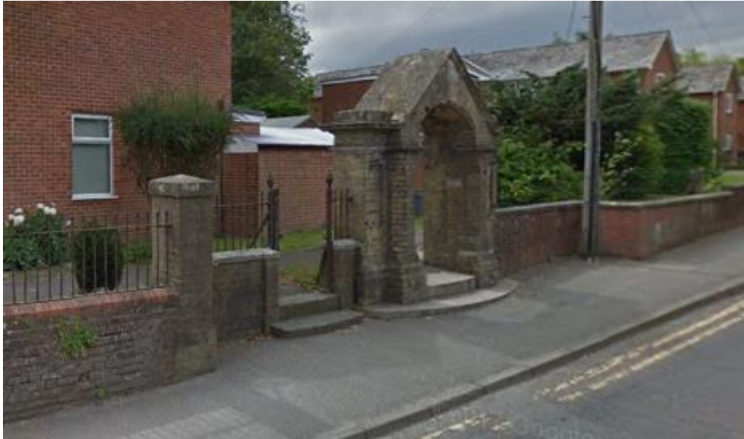
Plate 28. The former school entrance, wall and railings, Damory Street.
