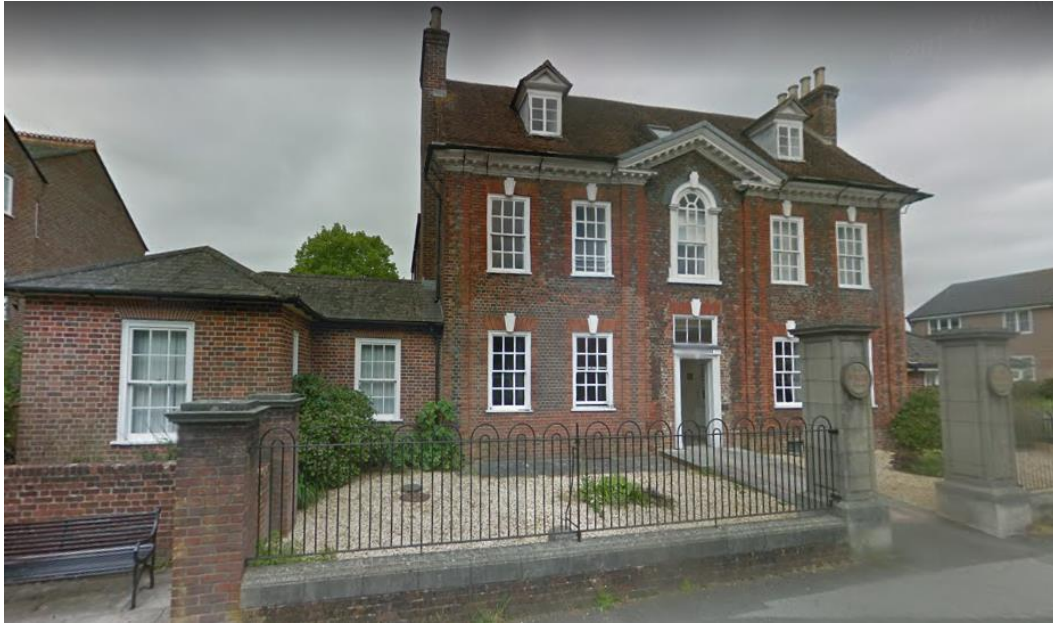
Plate 12. Eagle House, White Cliff Mill Street.
