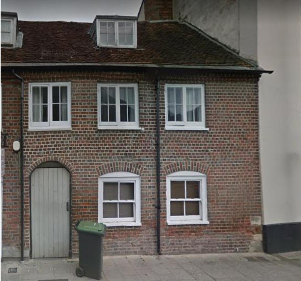
Plate 11. Fourth rate housing. Of particular note is the band of brick headers between ground and first floor windows. A similar approach can just be seen on the adjacent property to the left of the image.
