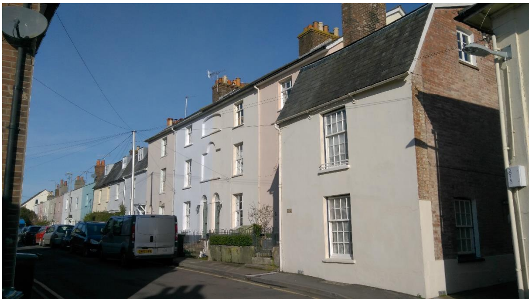
Plate 20. Higher and lower status 19 th century buildings in Orchard Street. Note the extensive use of render in contrast to the earlier taste for brick.
