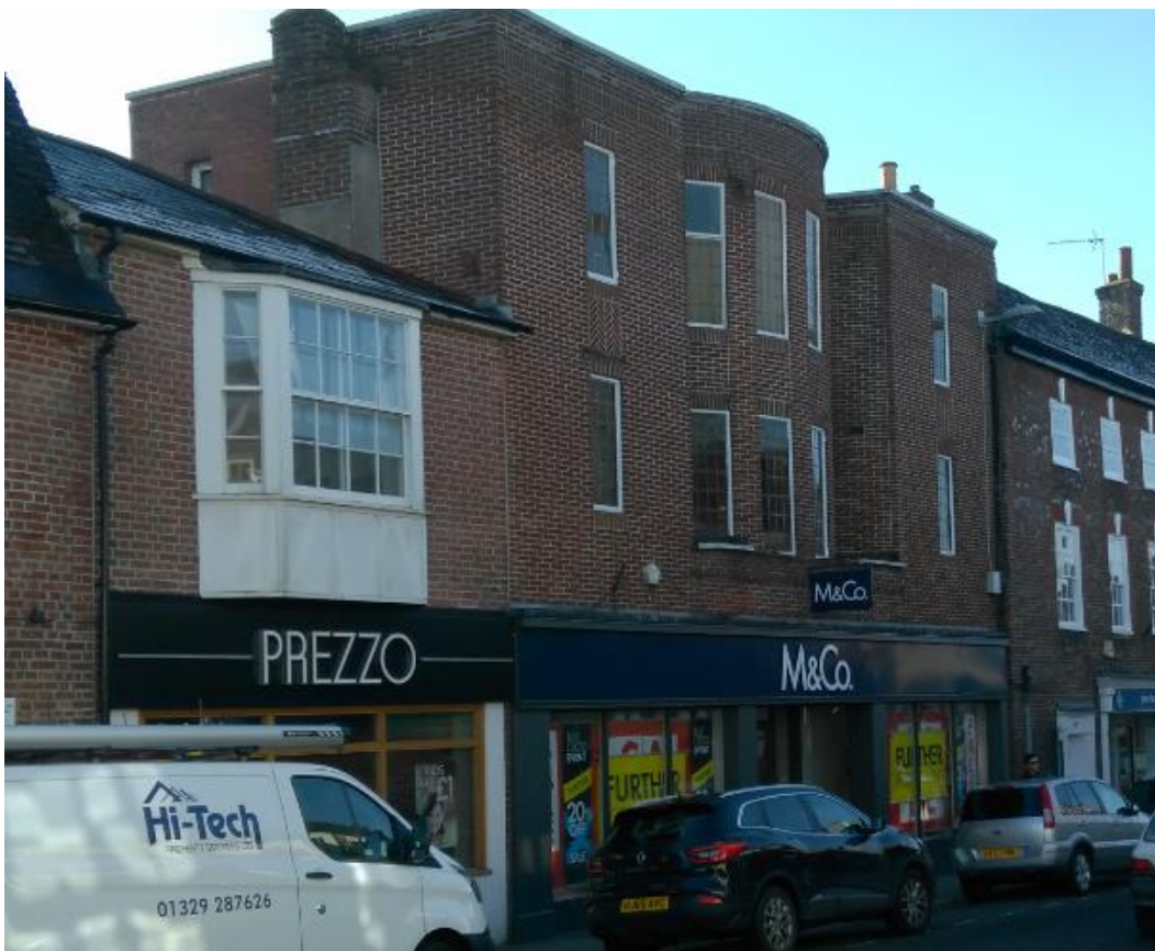
Plate 26. The former cinema, East Street.
