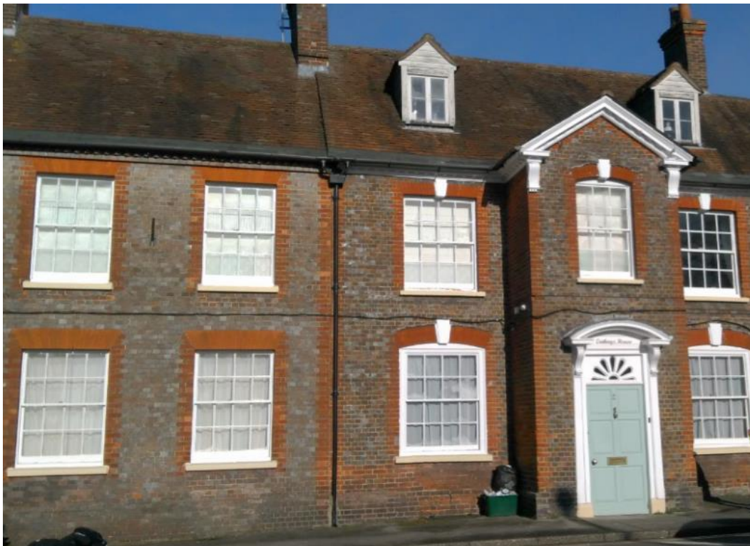
Plate 23. Typical 18 th Century materials, red brick with vitrified headers, clay tiled roof and timber windows, in this case vertical sliding sashes.
