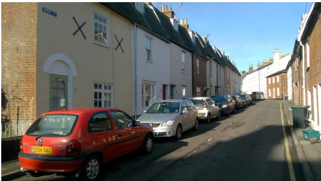
Plate 14. Lower rate 19 th century housing in Dorset Street. This level of housing has perhaps been subject of the most significant changes as a result of permitted development allowances.
