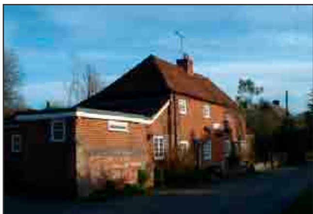
Whitsbury - the only significant settlement in this character area. Red brick is a common building material.
