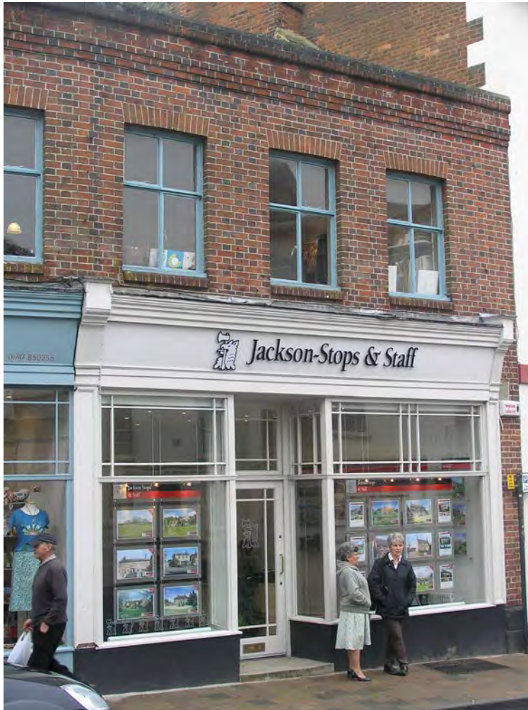
A good Art Deco (first half of the 20th century) shopfront in Shaftesbury with sensitive use of lettering and image on the fascia
