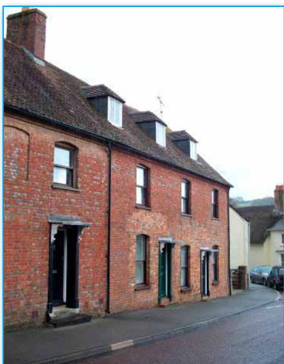
Dormer windows. Careful compositions using hipped roof dormers in Bere Regis and Corfe Castle.
