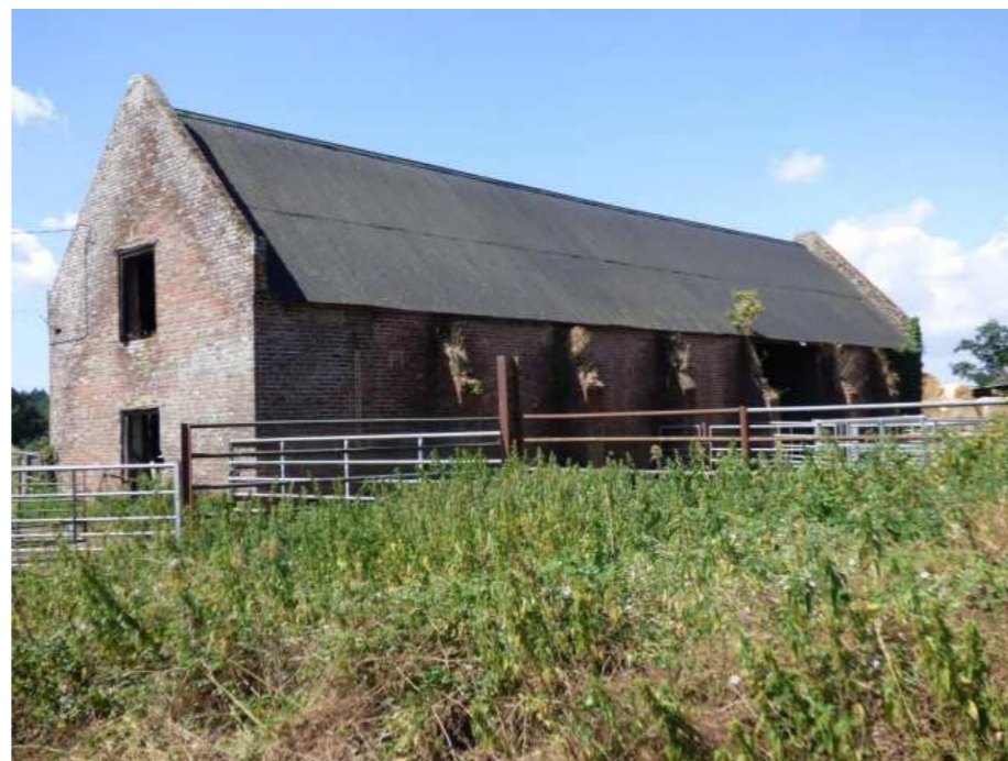
Plate 10. Philliol's Farm (Listed) Barn (facing NW)
