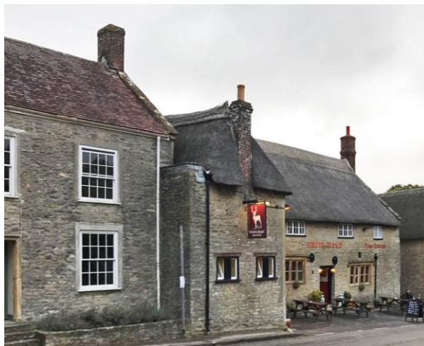
Photo: Yetminster High Street showing varying rooflines
