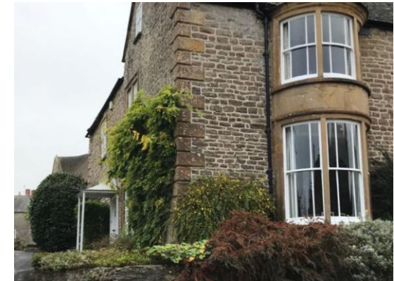
Photo: Junction of Queen Street with the High Street, Yetminster, showing corner treatment with windows on both sides
