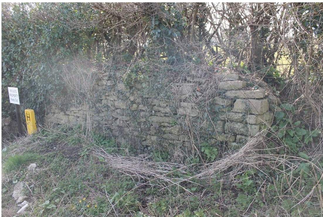
Plate 14. Former cottages at The Elm
